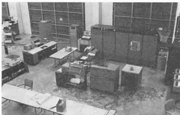
Figure 8. Lab GLC's Installed and Connected
