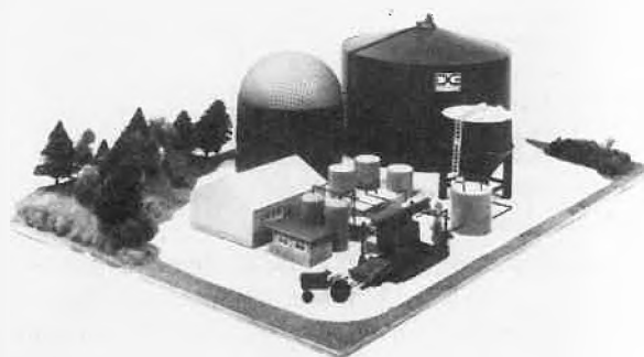
Fig. 1: This scale model is of an effluent treatment plant based on the Anox system now under construction in northern France.
