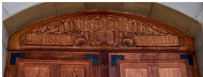
The door at Rämistrasse 76 still bears witness to the chemical history of the building. © Cristina Nevado.
